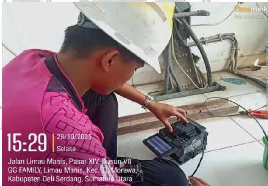
Figure 3 Splicing Cable of FO
