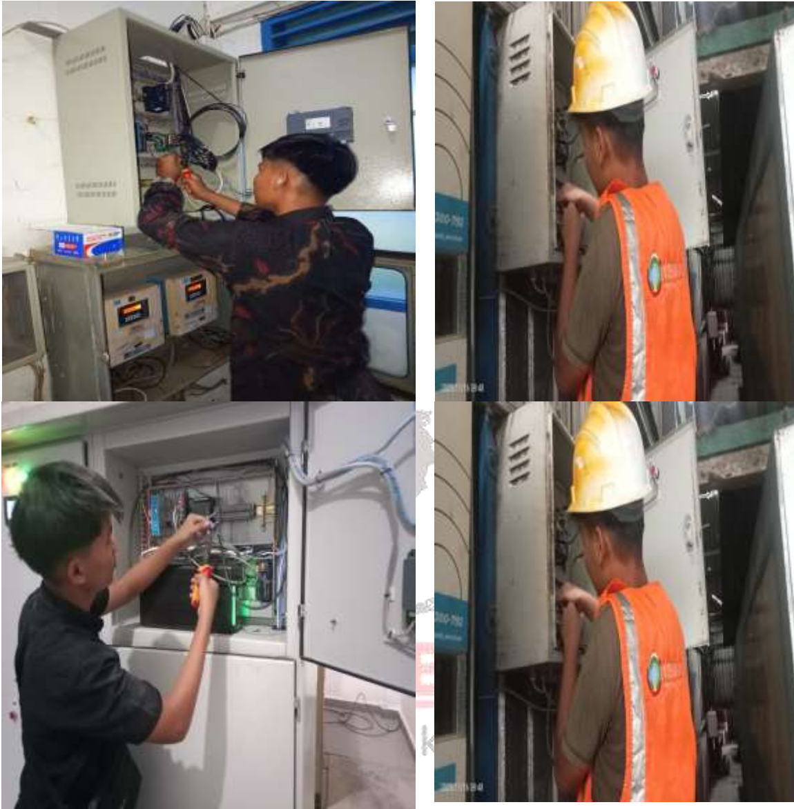
Figure 4 Cable Repair on Panel
