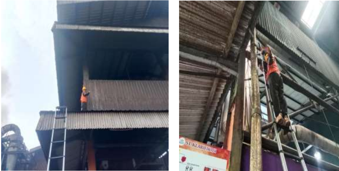
Figure 1 Pulling Analog Cables and FO Cables
